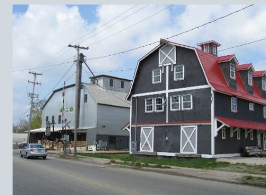
East Bridge Street
