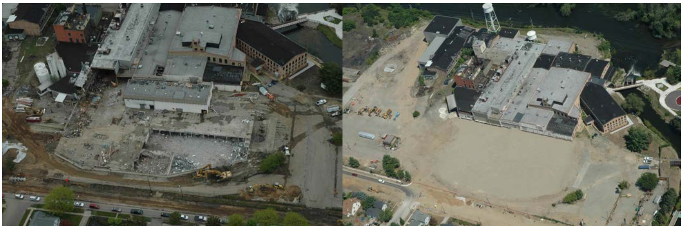
Mill building demolition in 2012, during and after.
