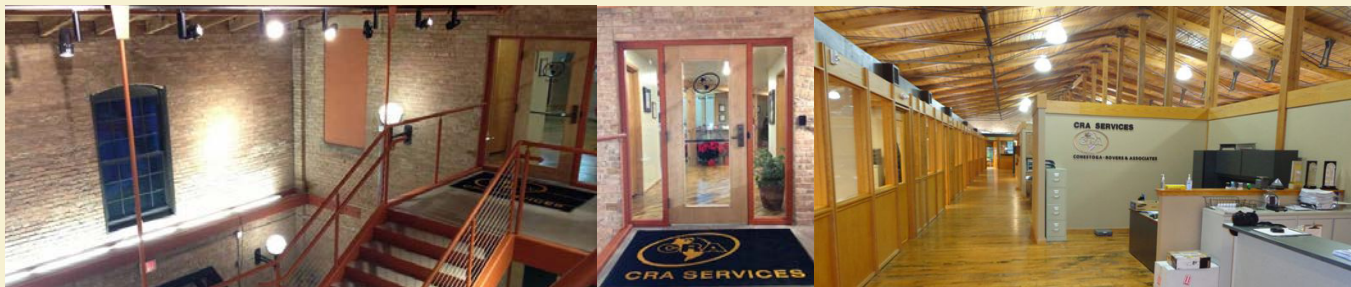
Adaptive reuse of the historic Plainwell Paper Mill.
