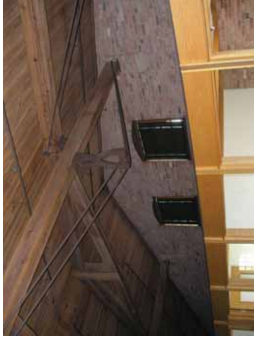
Timber Roof Structure Typical in Older Buildings on the Site
