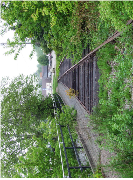
Railroad Bridge Over Mill Race
