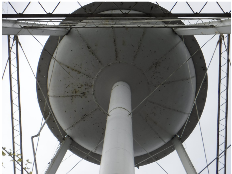
11) The bowl is in good condition. The coating is in poor condition.
