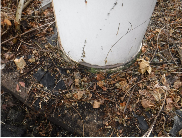
4) The riser foundation is in good condition.
